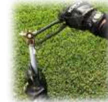
Tightening 9/16" 5/8" & 3/4" fuse nuts
